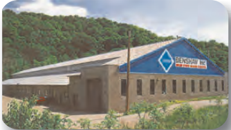
BENSHAW Inc. Plant2 Manufacturing Glenshaw, PA
