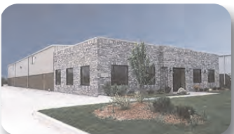
BEN-Tech Industrial Automation Rochester Hills, MI
