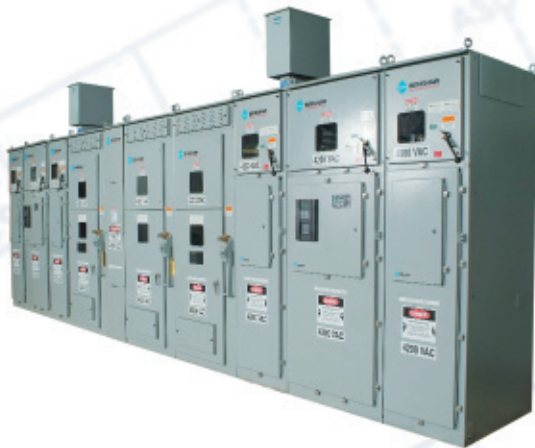
FUSED DISCONNECT MTM 7.2KV motor control center with integrated power factor correction
